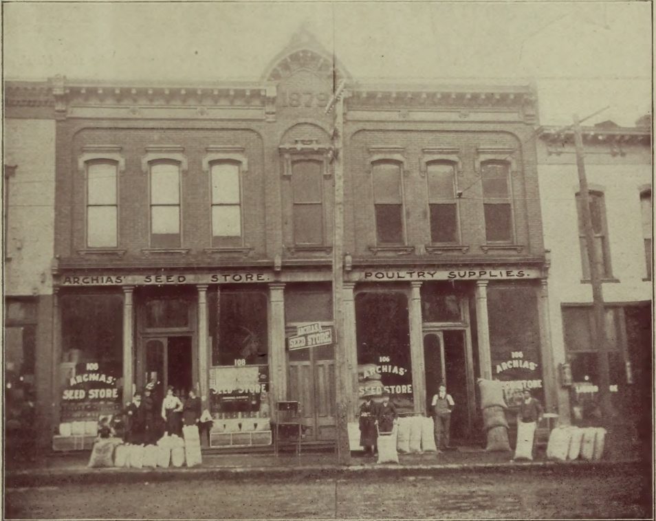
Front View of Our Seed Stores, 106-108 E. Main St., which have over 11,200 Square Feet Floor Space.
